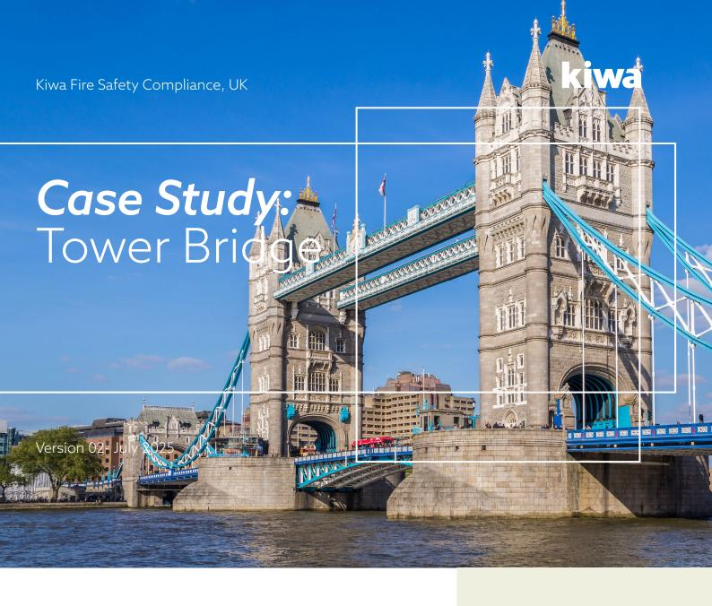
Tower Bridge (a grade 1 listed structure) is a combined bascule (a moveable bridge with a counterweight) and suspension bridge built between 1886 and 1894. The bridge crosses the River Thames close to the Tower of London and has become an iconic symbol of London. The suspension bridge deck connects the two towers and is freely accessible to both vehicles and pedestrians; whereas the towers, high-level walkways and Victorian engine rooms all form part of the popular Tower Bridge Exhibition.
